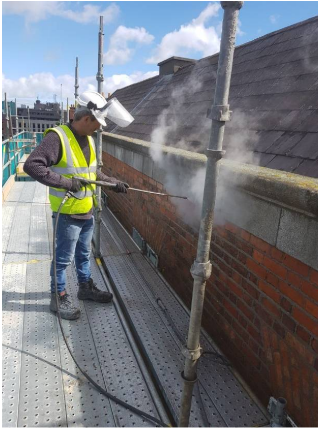
Steam pressure cleaning
