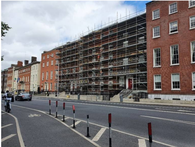
Scaffolding goes up July 2020
