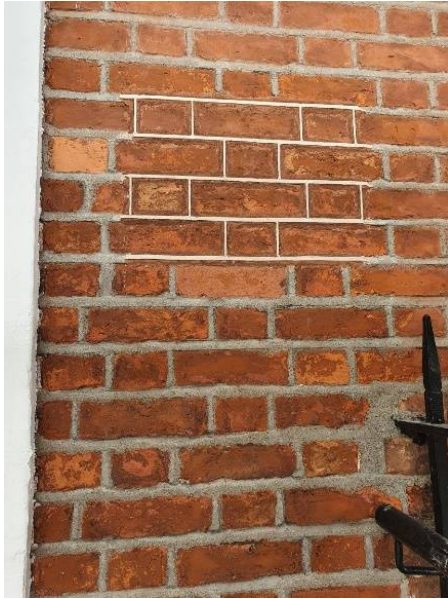
Old pointing with sample new section
